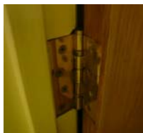
Morticed Hinge =
