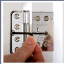
Adjust the hinge: Horizontally, To move the door side to side.
