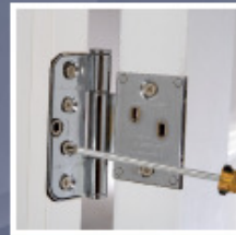
Adjust the hinge: Laterally, To move the door in and out.
